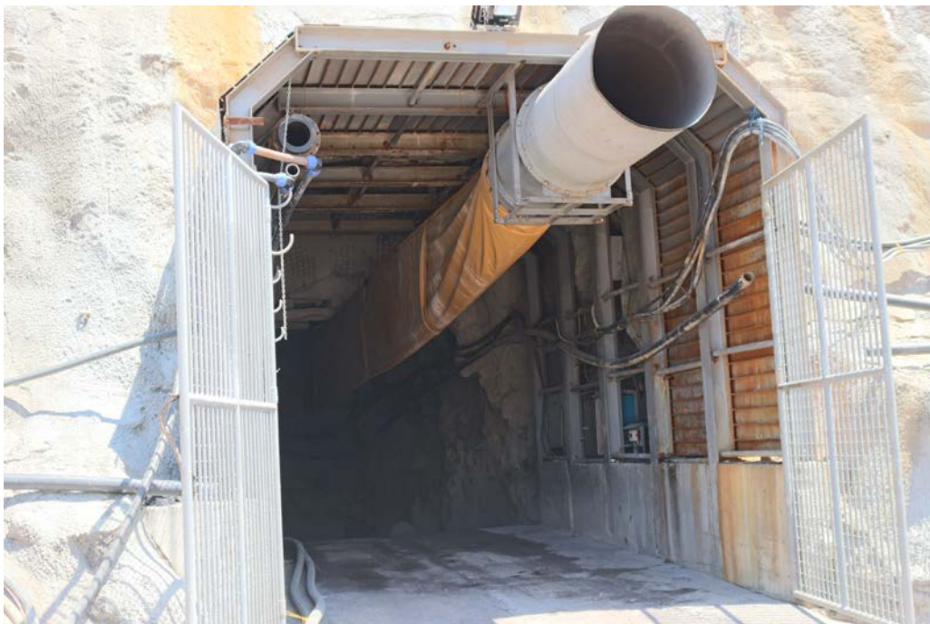
Figure 5: Portal to Main Access Decline
