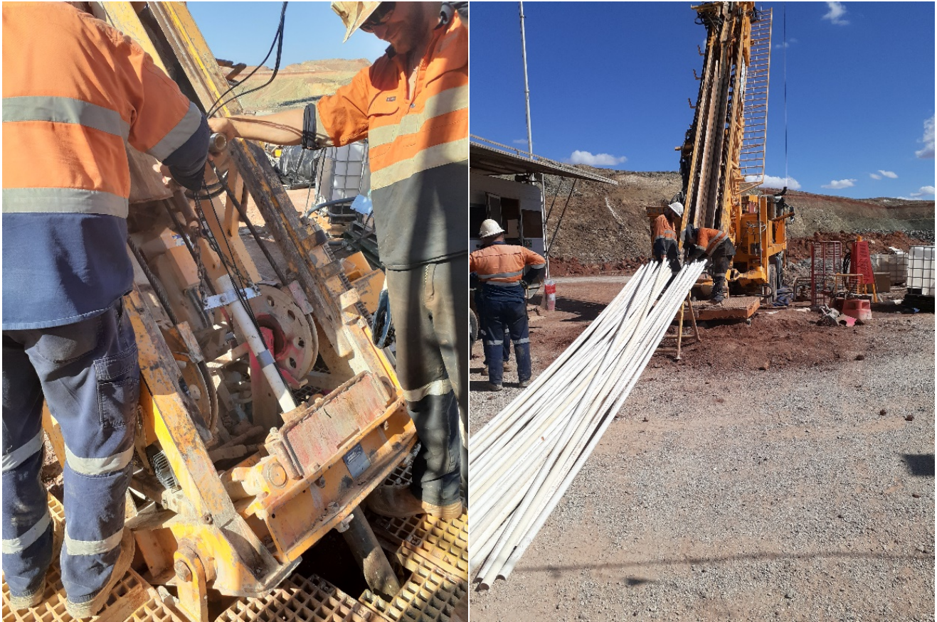
Figure 7: DDH1 installing vibrating wire piezometers in the KOTH open pit as part of geotechnical investigations.
