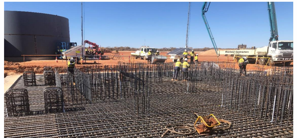
Concrete preparation for Mill base
