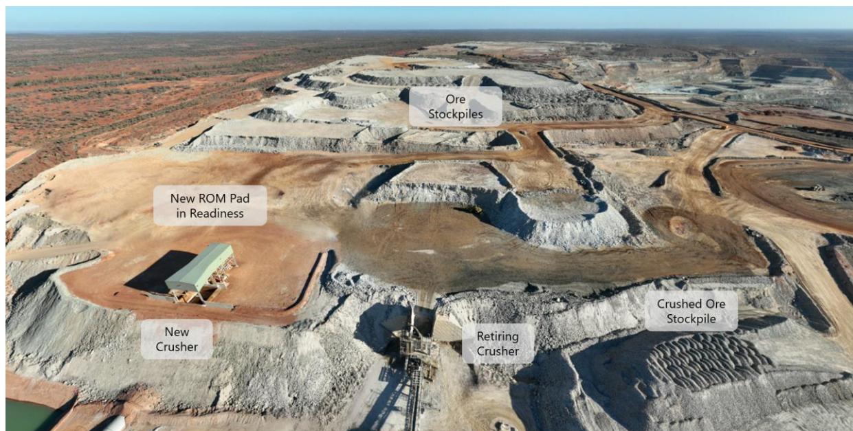
Figure 4: Crusher area and stockpiles
