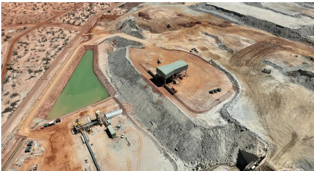
Figure 1: New crusher installation
