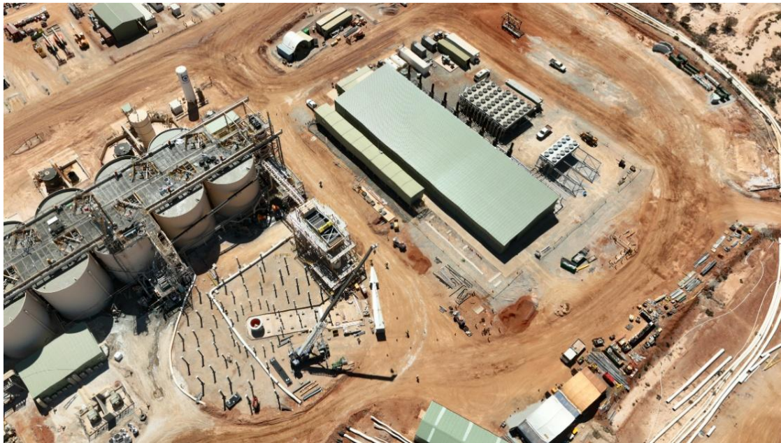
Figure 2: Stage 1 wet plant upgrade complete with 4 new CIL tanks online. Stage 2 works including a tailings thickener and powerhouse extension progressing well
