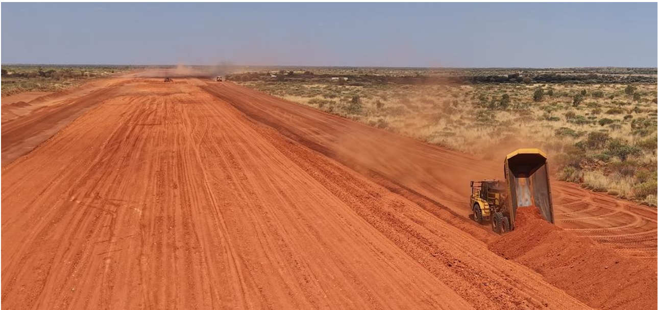
Figure 6: Construction of airstrip in progress
