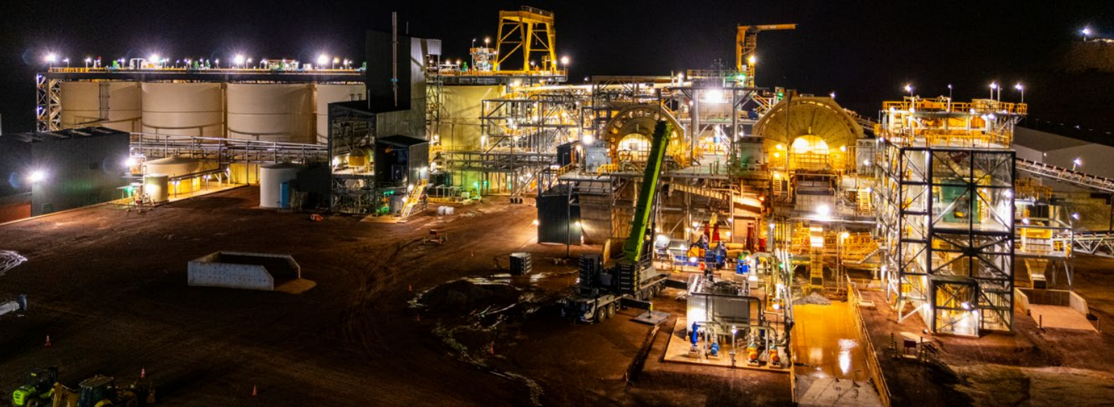
Kiaka process plant
