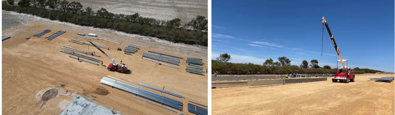
Figure 2. Structural steel arriving onsite in Wickepin
