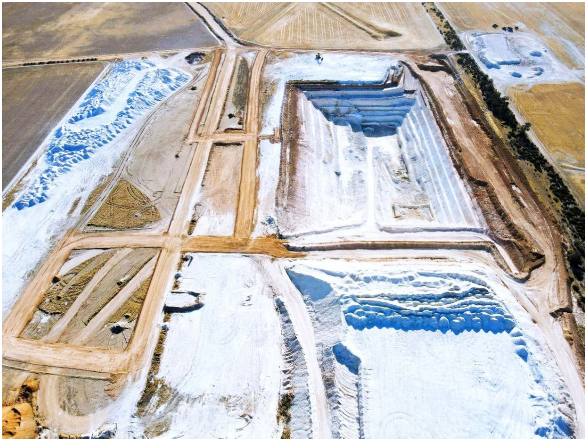
Figure 1: Aerial view of new roadways for Traffic Management System – 28 January 2026
