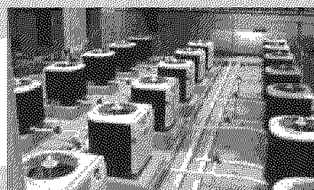
Focus Temp Heat Pump Installation
