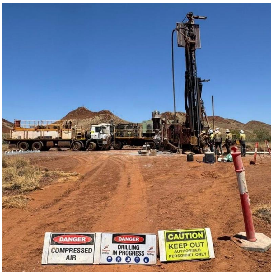
Figure 1: NexGen Drilling RC Drill
