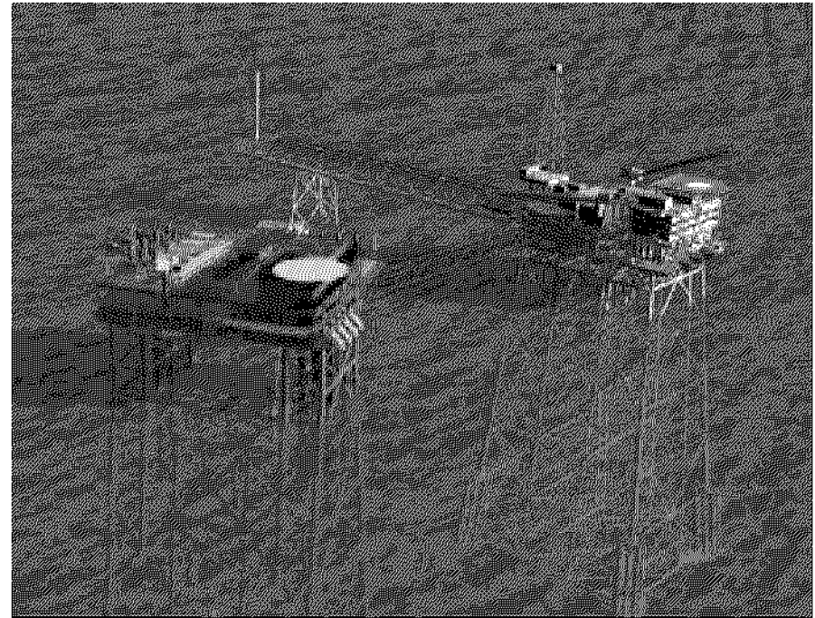
NRB Compression Platform Bridge Linked to NRA
