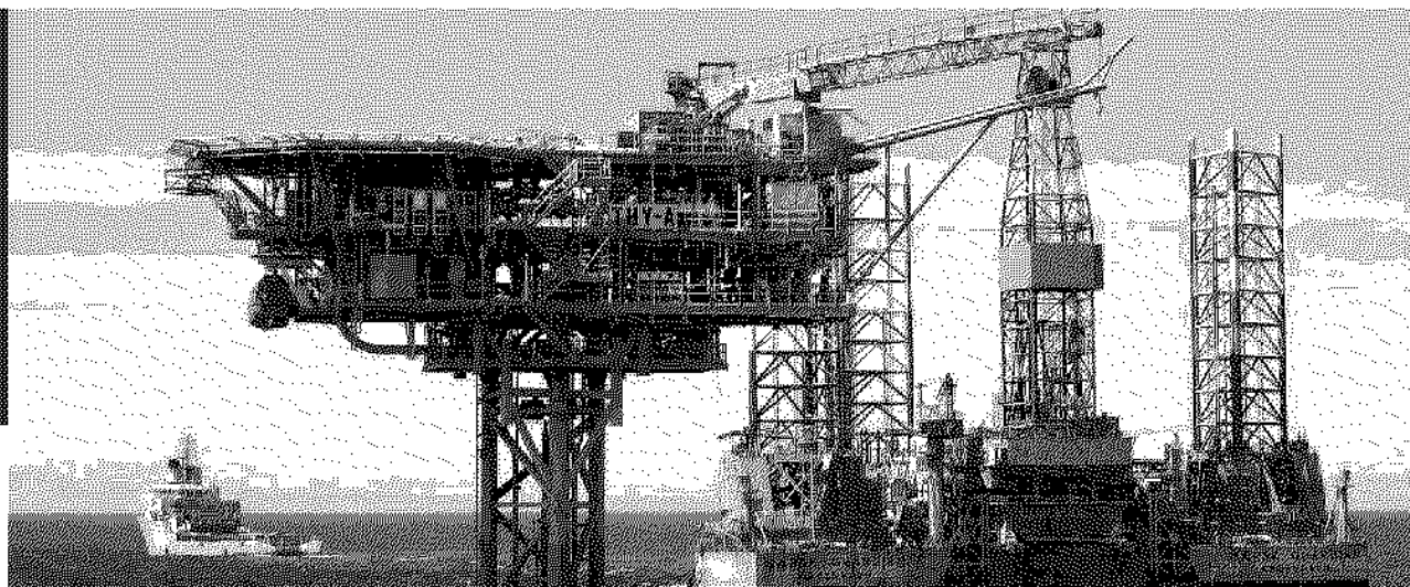
Otway's well head platform is the first remotely operated production facility for Woodside in Australia which will be operated by staff at the onshore plant's central control facility.
