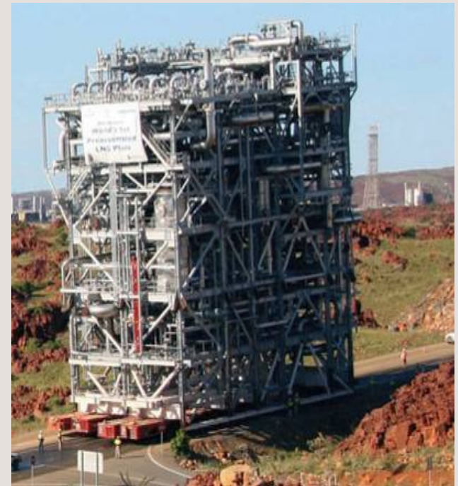
Train 5 liquefaction module on route to KGP, 2007
