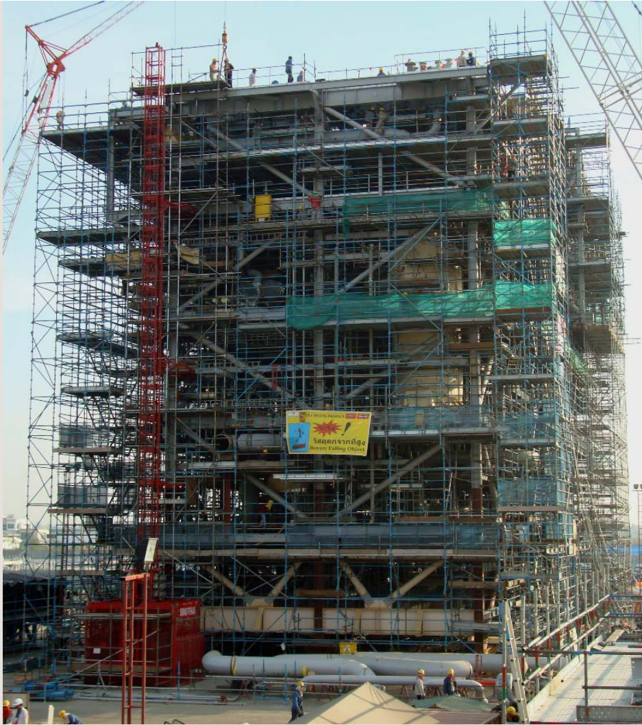
Pluto liquefaction module under construction at Laem Chabang, Thailand
