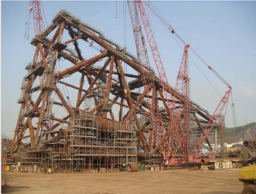
Pluto jacket under construction at Shenzhen Chiwan Sembawang
