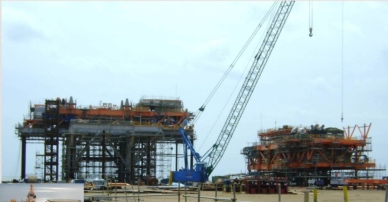
Pluto topsides construction in Ramunia, Malaysia
