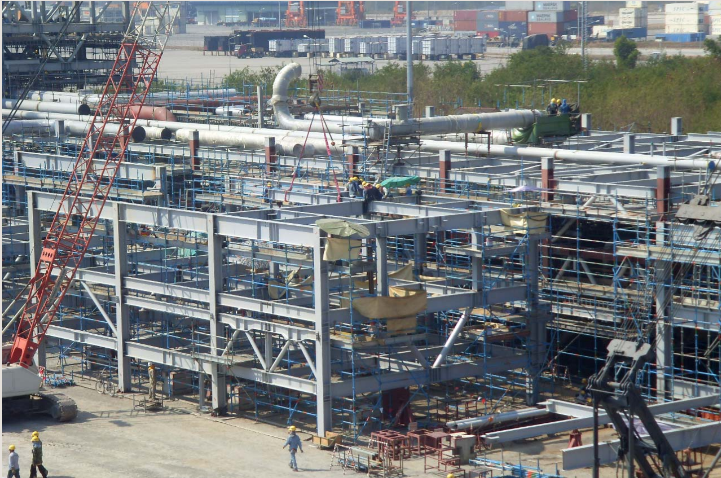
Construction at Laem Chabang, Thailand
