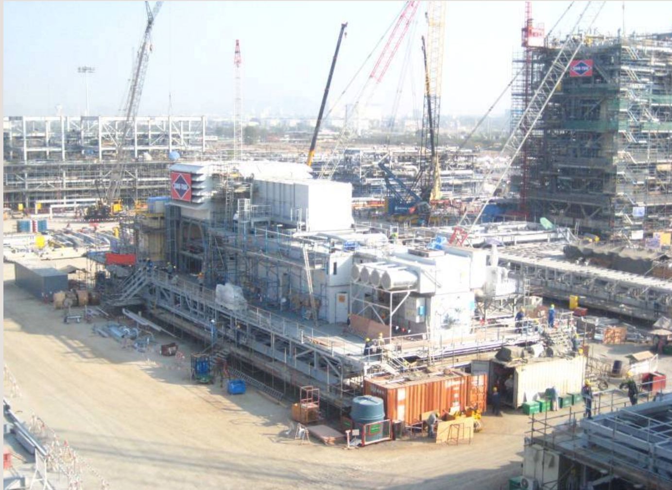
Gas turbine power generation unit under construction at Laem Chabang, Thailand
