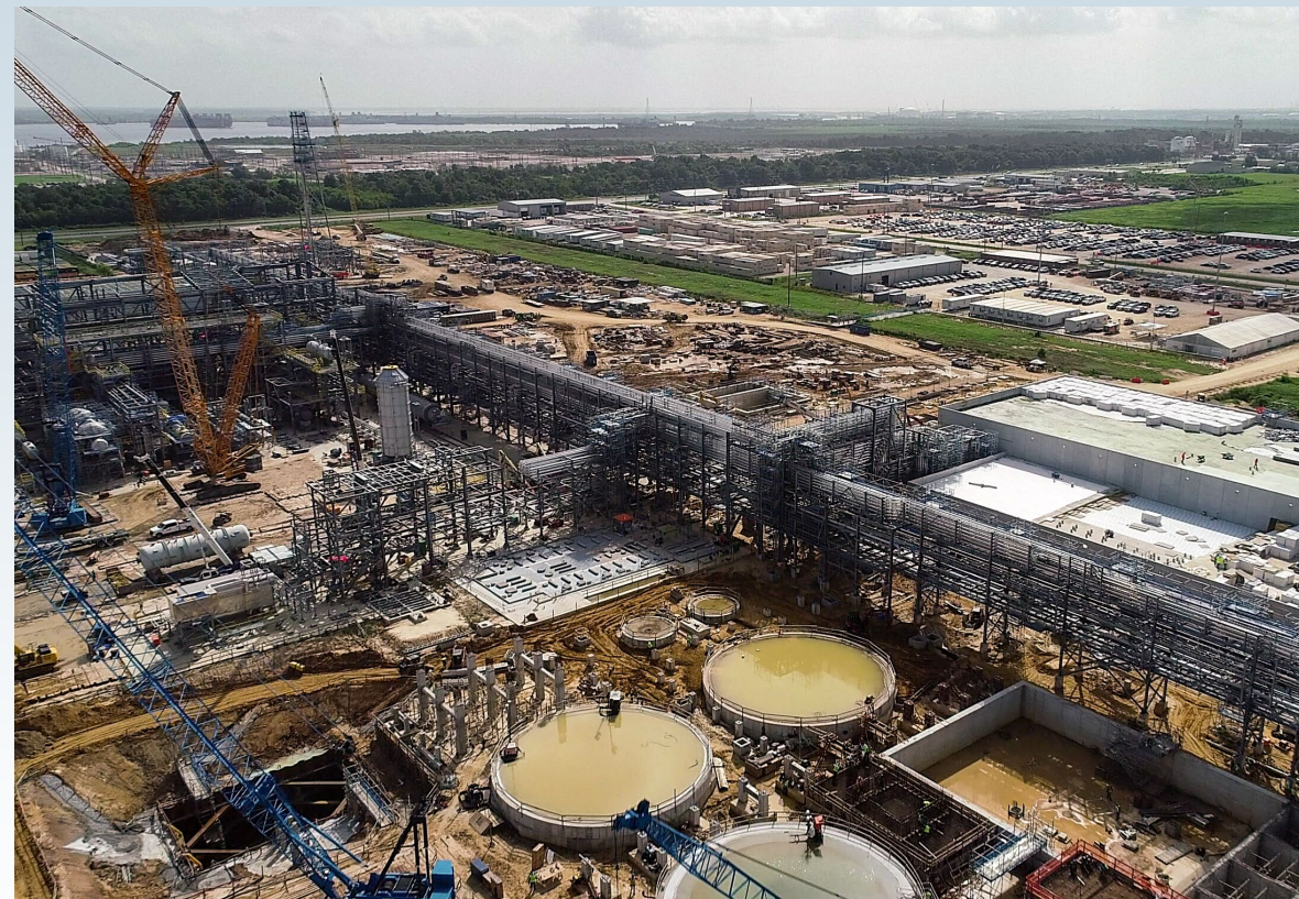
Beaumont New Ammonia Project under construction
