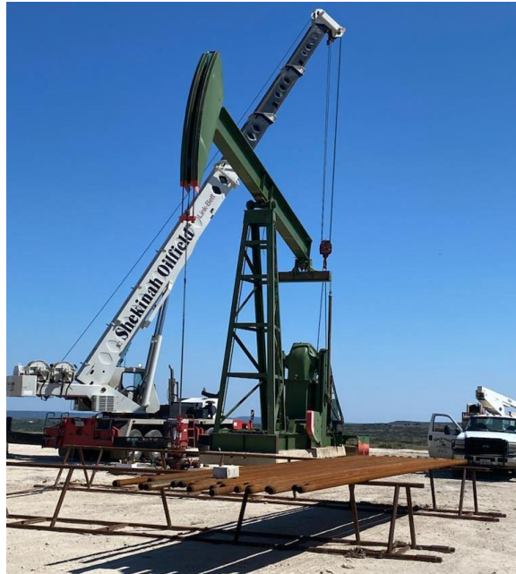
Figure 1: Pump installation at McLeod 1705
