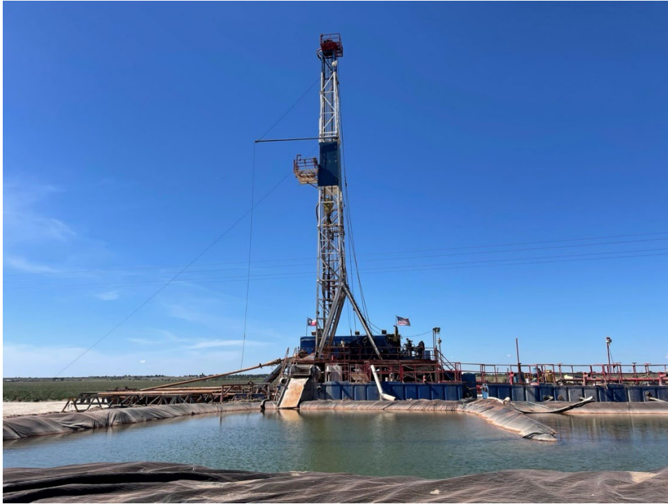
Photo 2. JVU-5 drill rig and lined pit.
