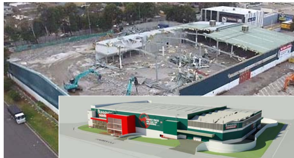
Caringbah, NSW store demolition & proposed new store
