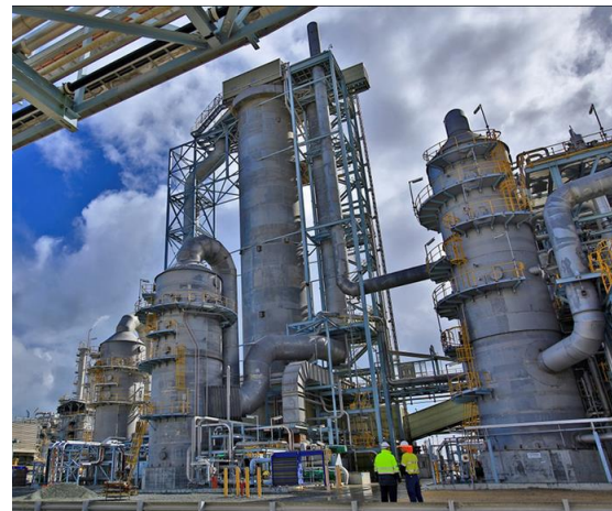
CSBP site at Kwinana, Western Australia
