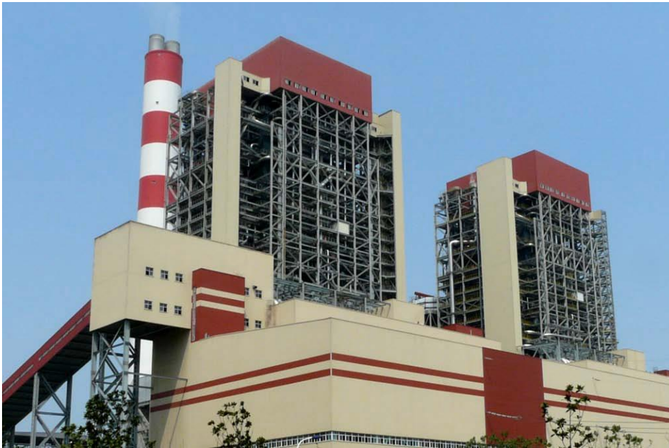
Waigaoqiao No3 Power Station
