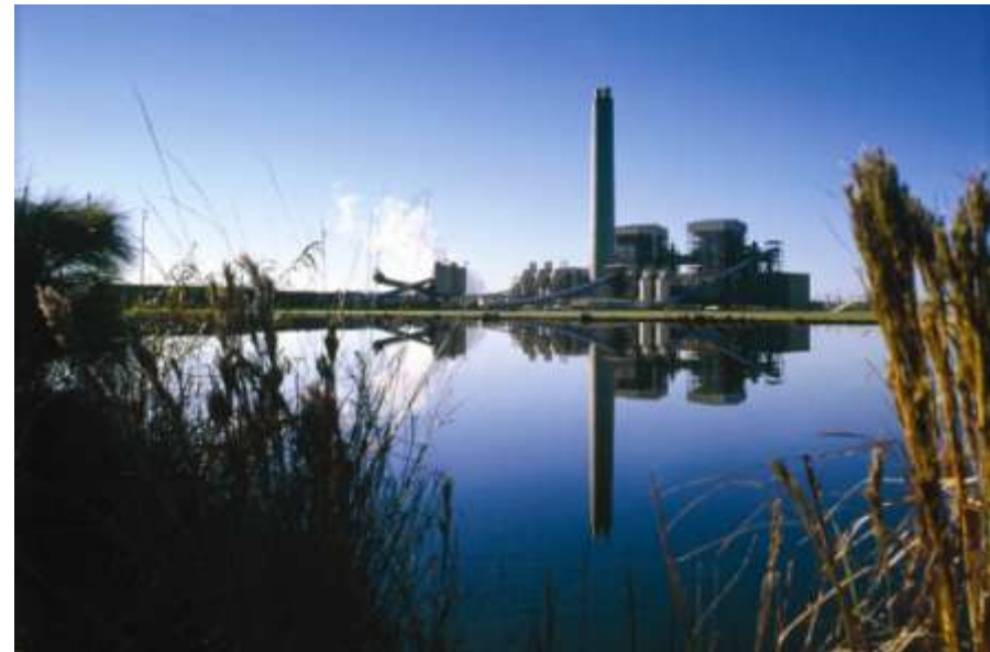
Santee Cooper – Cross Station Coal Fired Power Plant, USA
