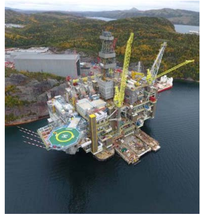
Completed Hebron topsides at Bull Arm, Newfoundland and Labrador (NL)
