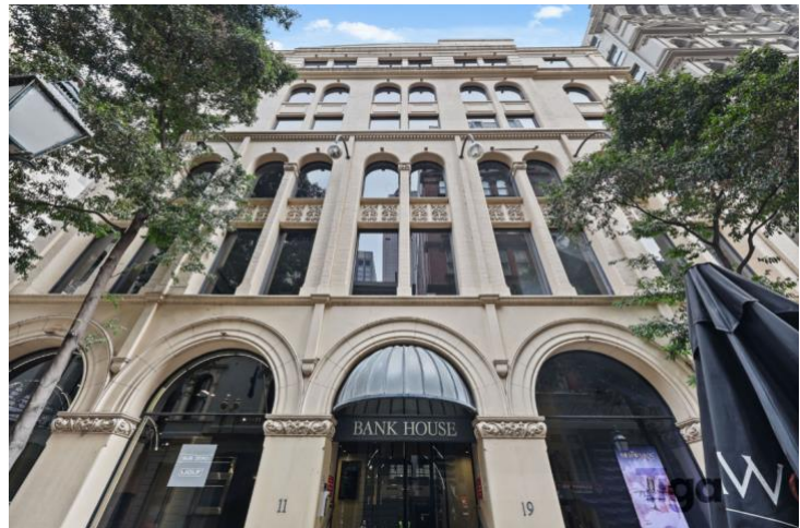
Bank House, Melbourne
