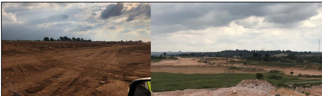
Image 4: Pit 2's rehabilitation completed during the quarter
