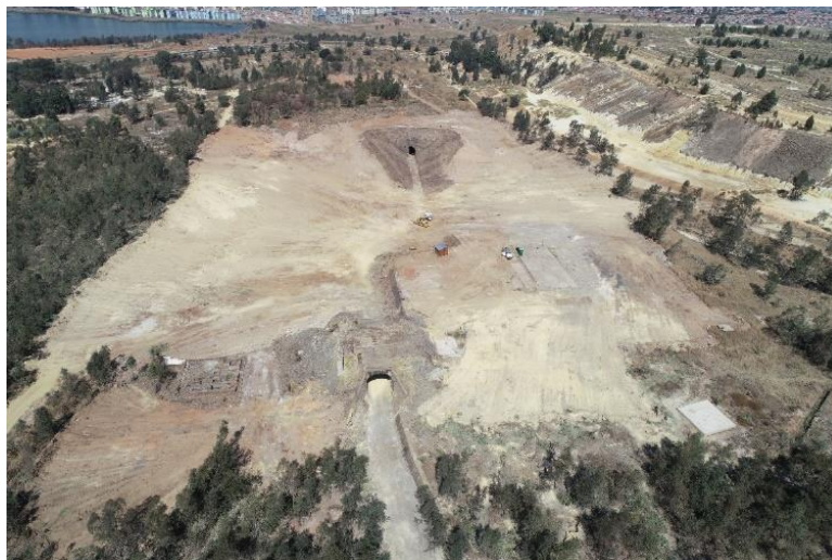
Image 1: Qala Shallows Site Preparation
