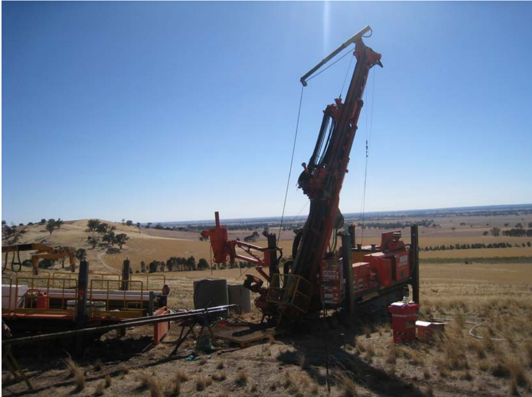
Figure 3 – Drilling geotechnical hole GTC2 at Golden Camel
