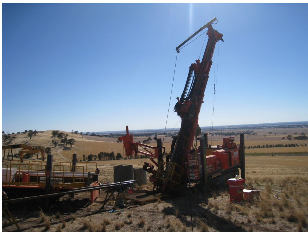
Figure 3 – Drilling geotechnical hole GTC2 at Golden Camel
