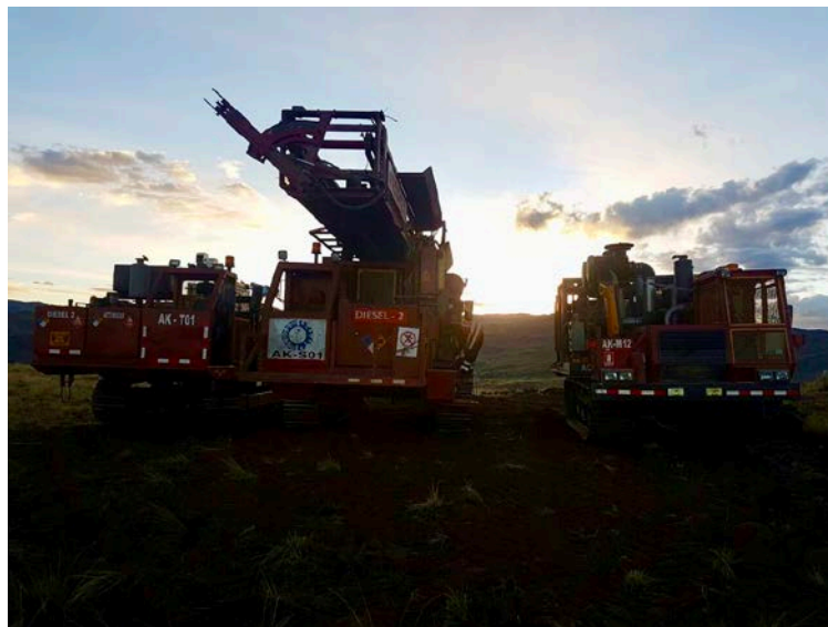
Drilling Rig & Equipment at Berenguela
