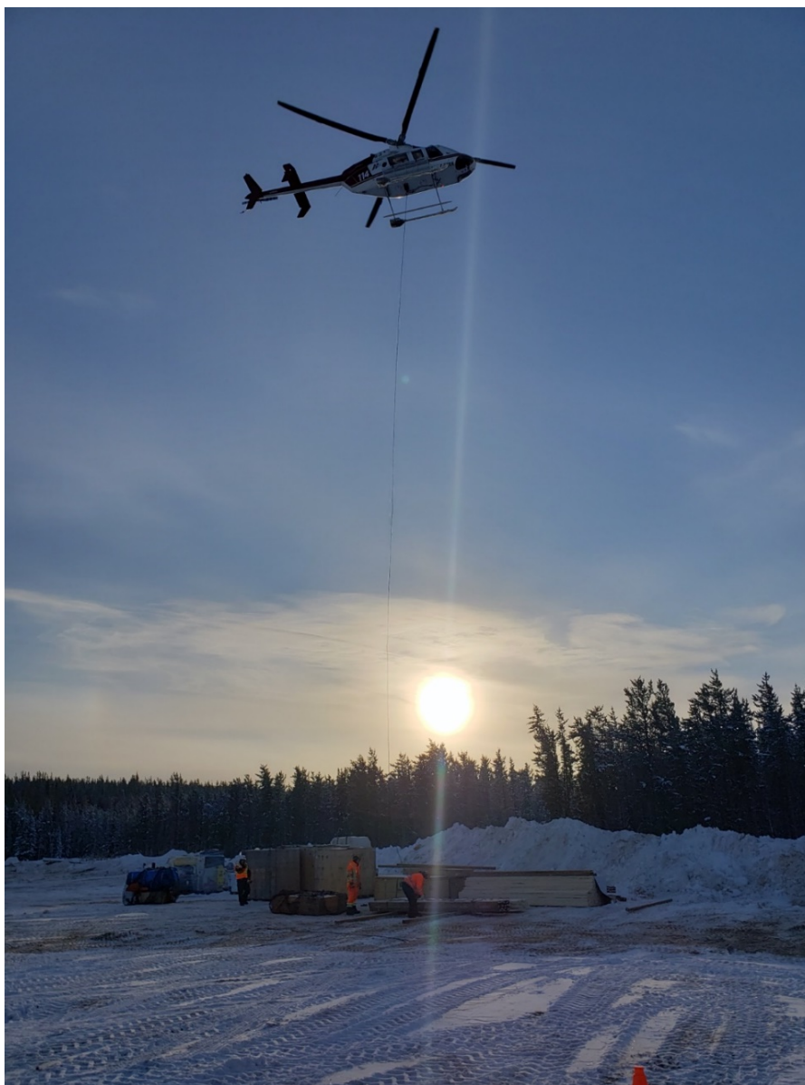
Figure 1: Helicopter Transport Services' Helicopter at Laydown Yard – Camp Construction
