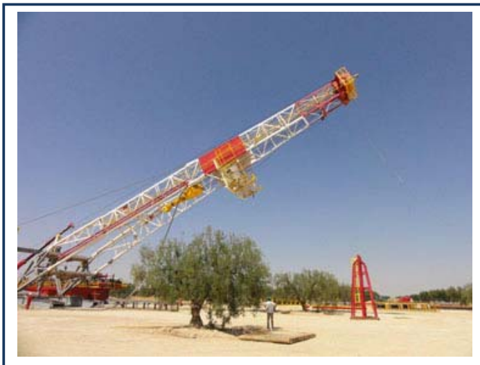
Figure 1: Sidi Dhaher Rig installation
