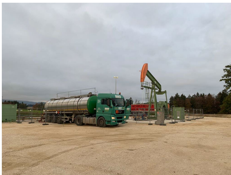
Oil tanker offloading at Anshof-3 location
