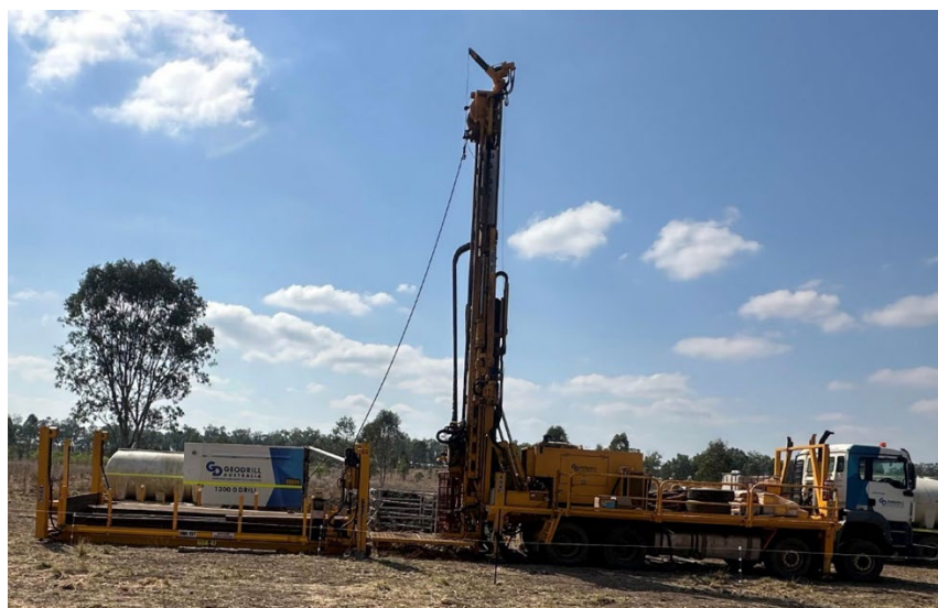
Figure 2: Drilling rig on site at the Rolleston South Coal Project
