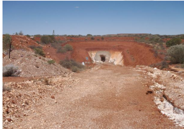
K2 Box-cut and portal
