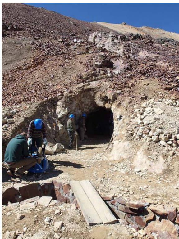
Figure 2: Re-opening Española 1 4805 adit
