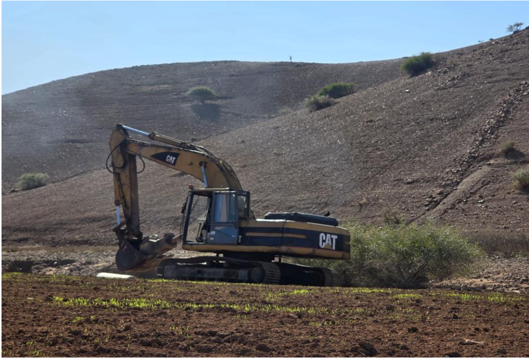
Figure 1- Excavator Mobilised to Site
