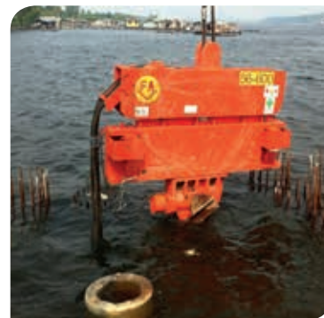
Offshore Vibratory Piling
