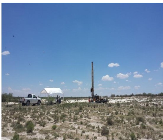
Shallow Auger Drilling at San Juan Project
