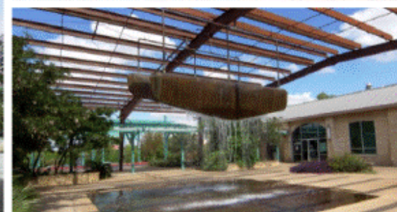
3601 South Congress- Existing Buildings
