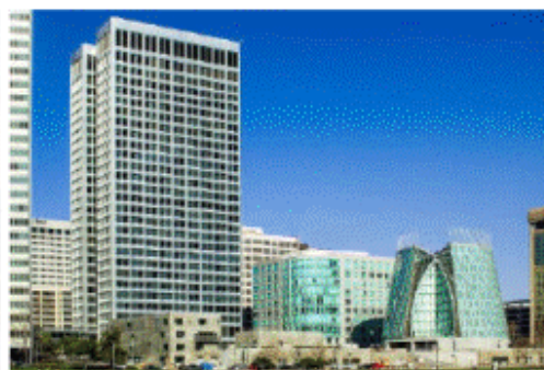
1 Kaiser Plaza – Existing Building
