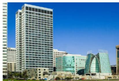
1 Kaiser Plaza – Existing Building
