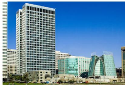
1 Kaiser Plaza – Existing Building
