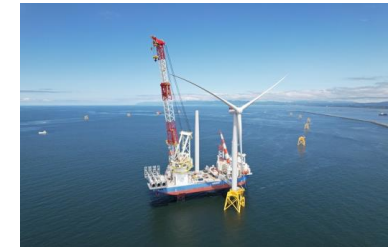
<Turbine Generator Installation>
