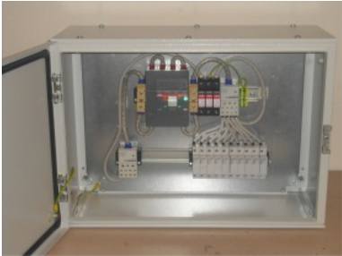
Figure 3: Board of Parallel Strin
