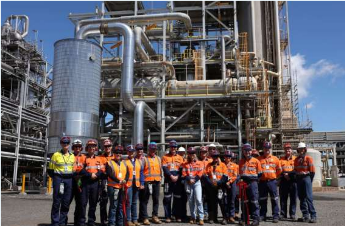
Official opening of Nitrous Oxide Plant, April 2024
