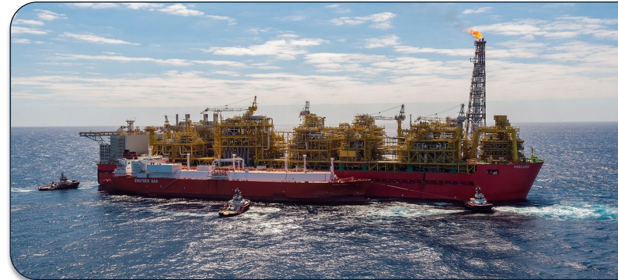
Prelude Floating Liquefied Natural Gas (FLNG) facility
