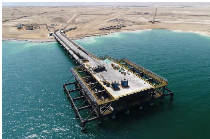
Photo 13.1: DSW Pumping station P9
