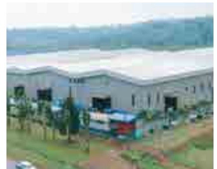
6 Ajiya Safety Glass Sdn Bhd Segamat, Johor
