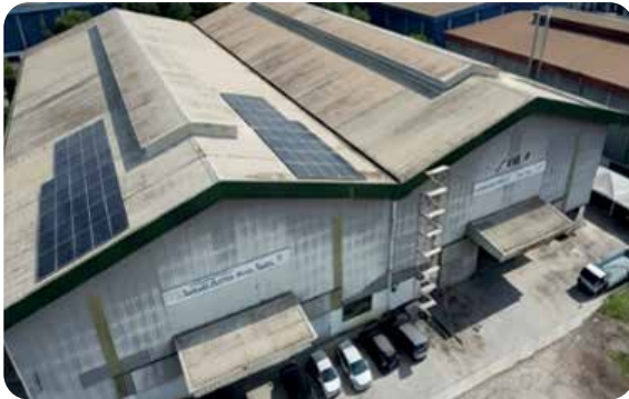
Solar PV Installation, Johor.
