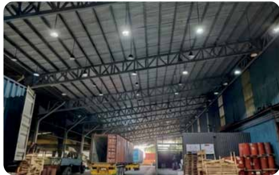
100% LED Lighting Transition.
