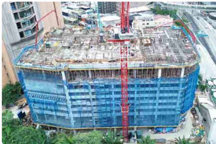
TS2 project construction progress.
