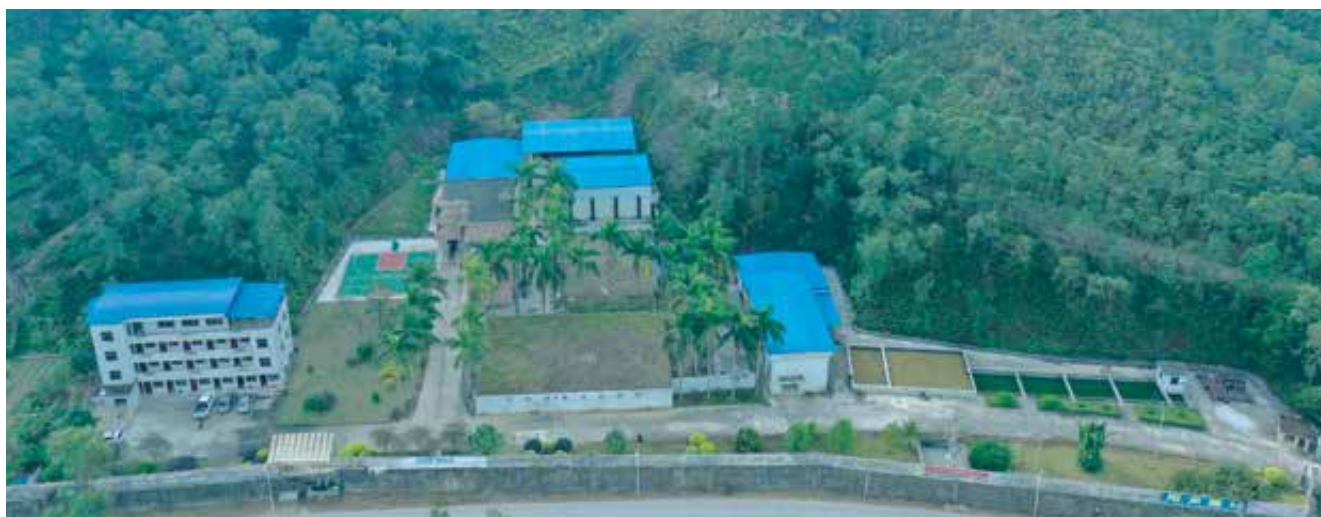
The Boluo Longxi water treatment plant in China
