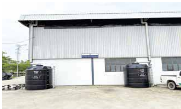
Rainwater tank for general purposes
