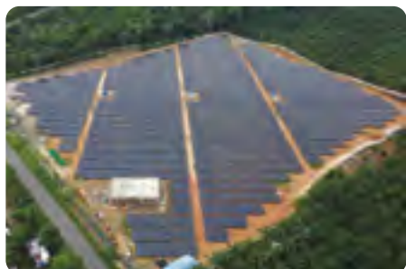
Large-Scale Solar Project, Tawau
